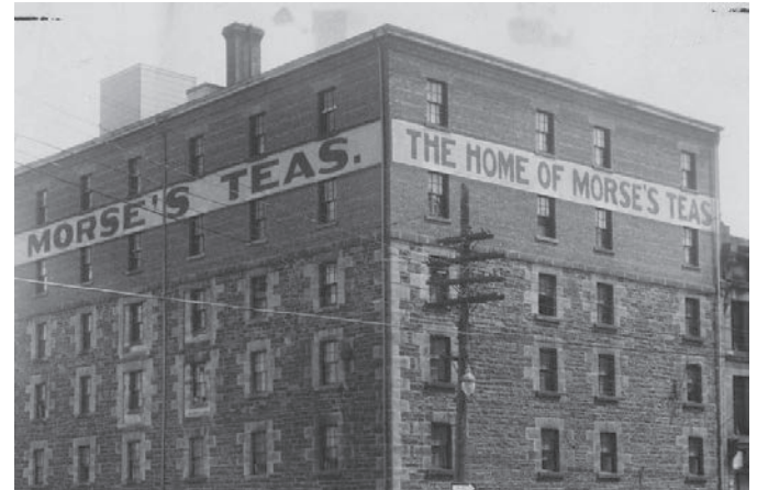
Figure 17. Photograph showing the appearance of the Morse's Teas Building following the renovation 9 .
