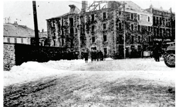
Figure 16. Image showing damage to the building 8 .
